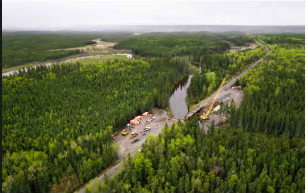
Construction crews replace a bridge along the Hudson Bay Railway.
