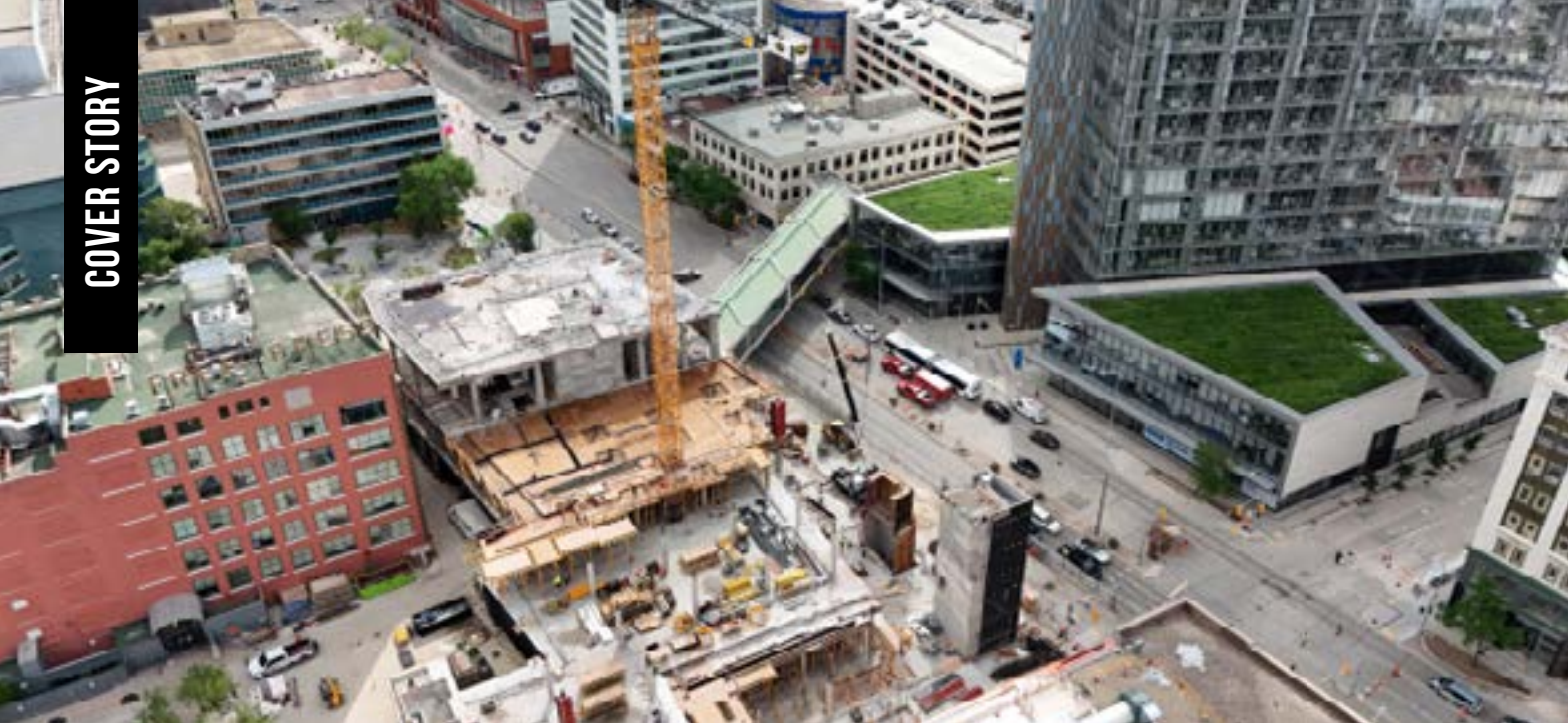
A photograph captured by drone shows the construction site and crane, which was erected in April.
